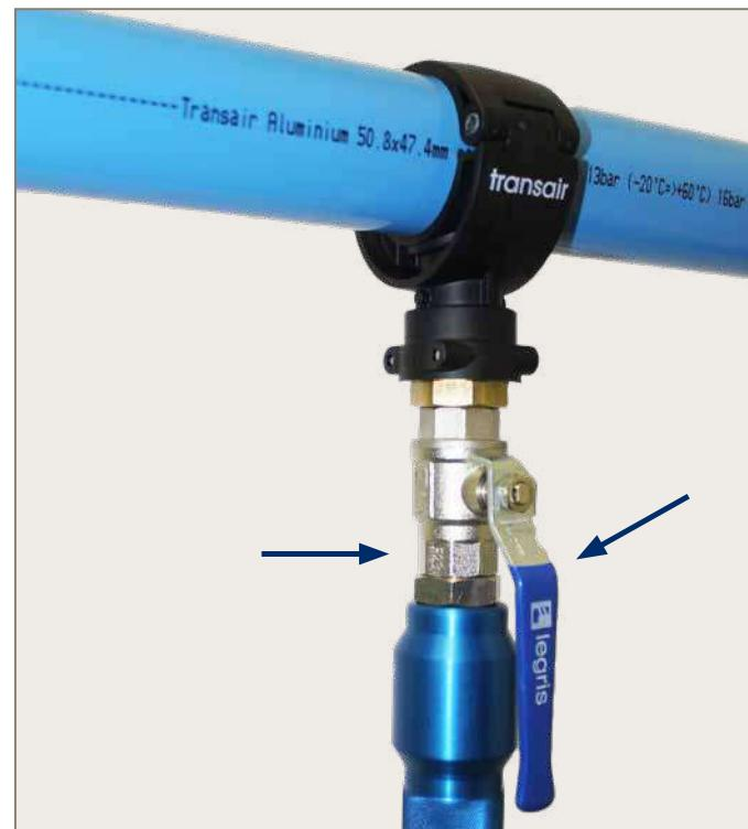
2. Thread the drilling tool onto the ball valve. Ensure the valve is open then fully drill the hole.
